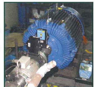
Right: Laser Alignment being performed prior to operational load testing
