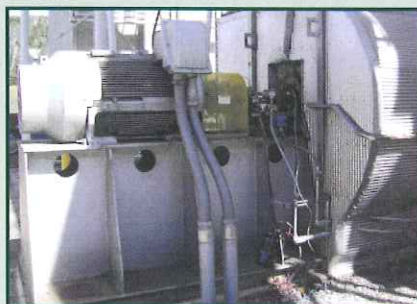
Right: On-site Dynamic Balancing of a large I.D. fan at a power plant
